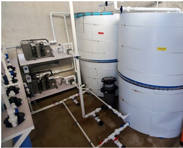
Figure 1. Seawater reservoir system
