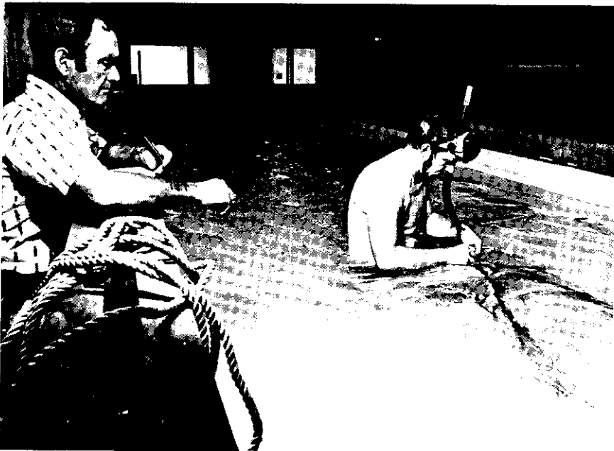
Fig. 2. Trawl model during test in Hydraulic flume.
