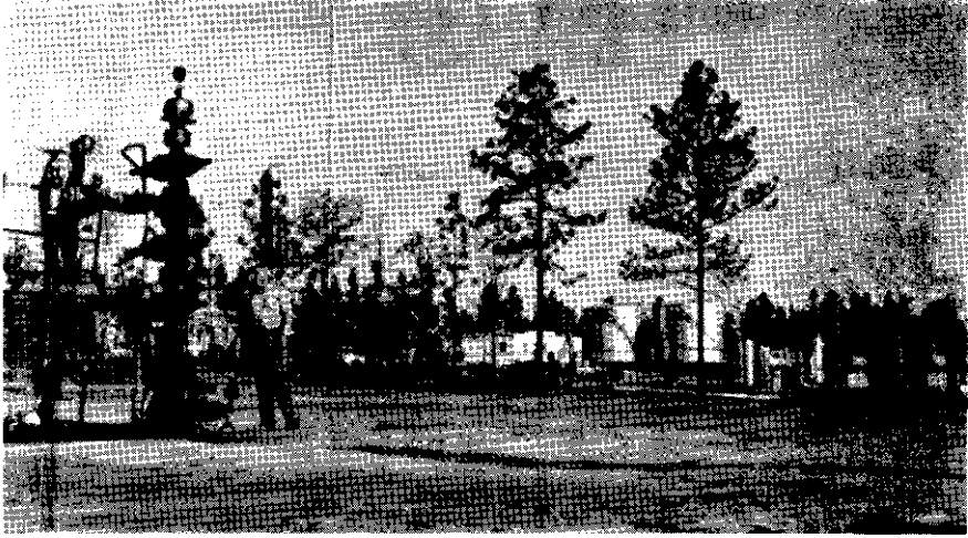
Fig. 4. Jay Field discovery well and plant.
